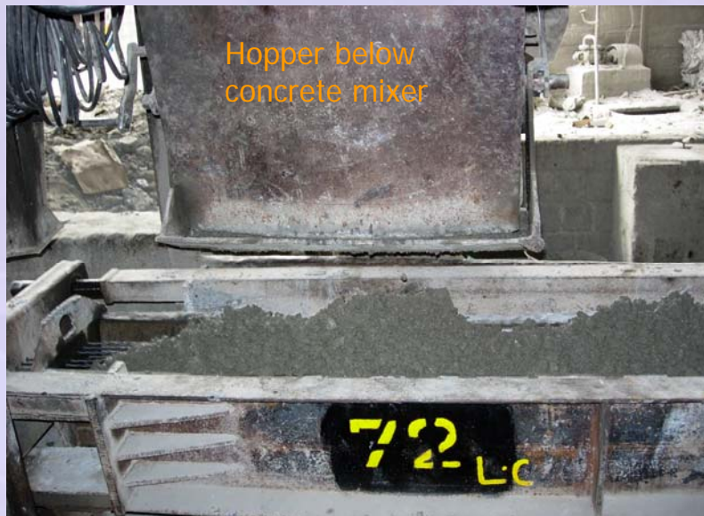
(g) Pouring of concrete
