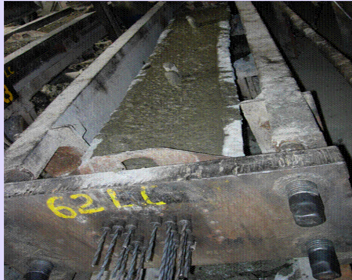
(h) Concrete after vibration of mould
