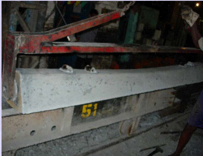
(k) Demoulding of sleeper
