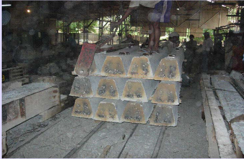
(l) Stacking of sleeper
