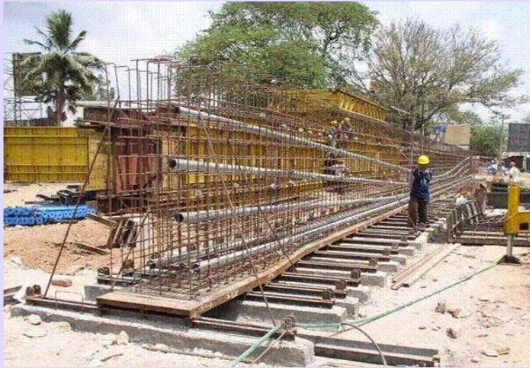
(a) Fabrication of reinforcement
