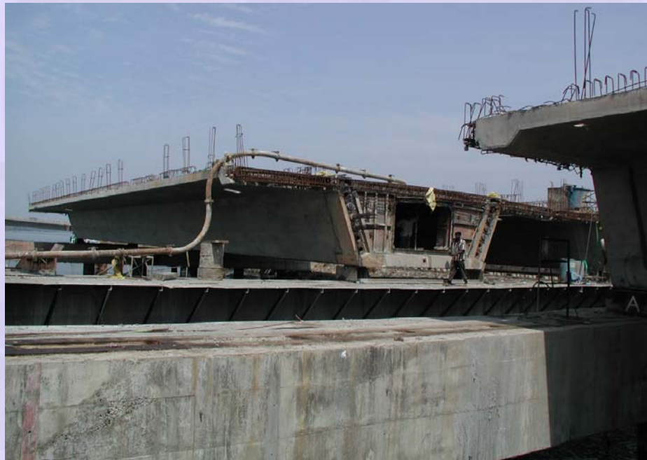
(c) Post-tensioning of box girder
