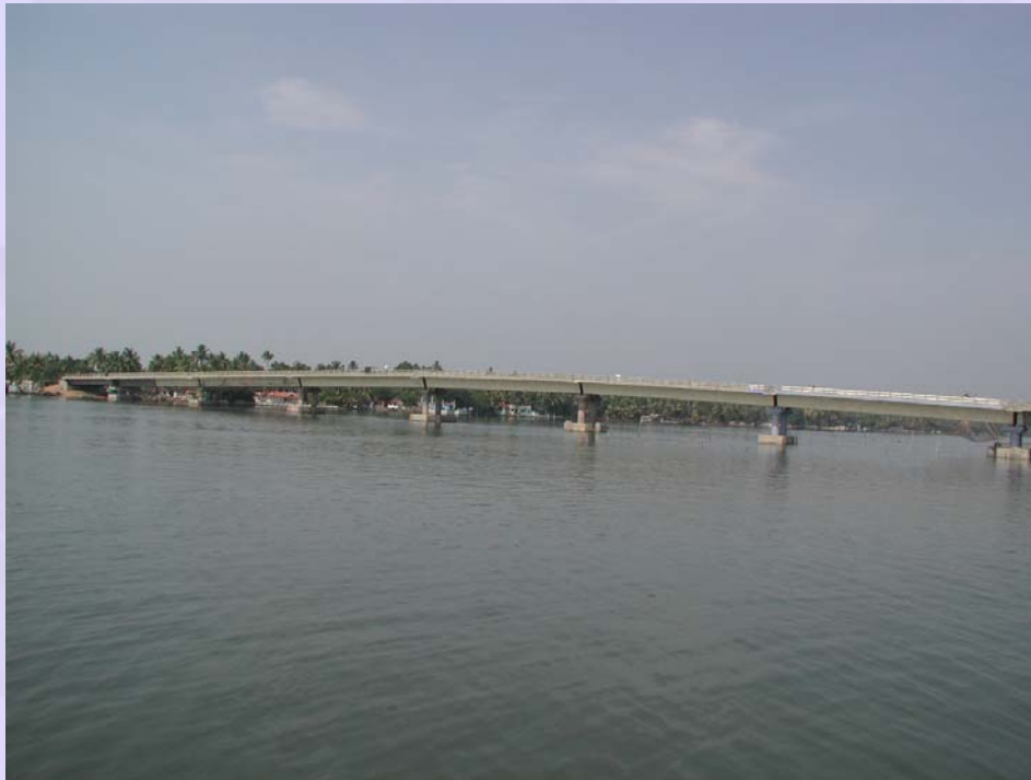
(e) Completed bridge
