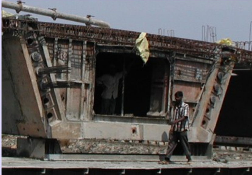
Figure 1-4.3 Post-tensioning of a box girder (Courtesy: Cochin Port Trust, Kerala)
