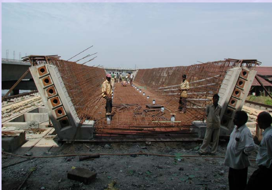
(a) Reinforcement cage for box girder
