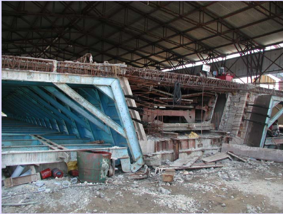
(b) Formwork for box girder
