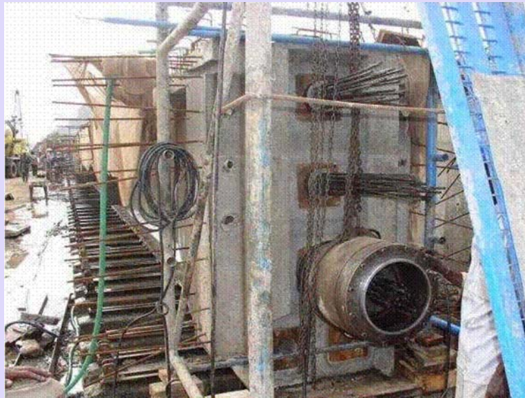
(c) Stretching and anchoring of tendons
