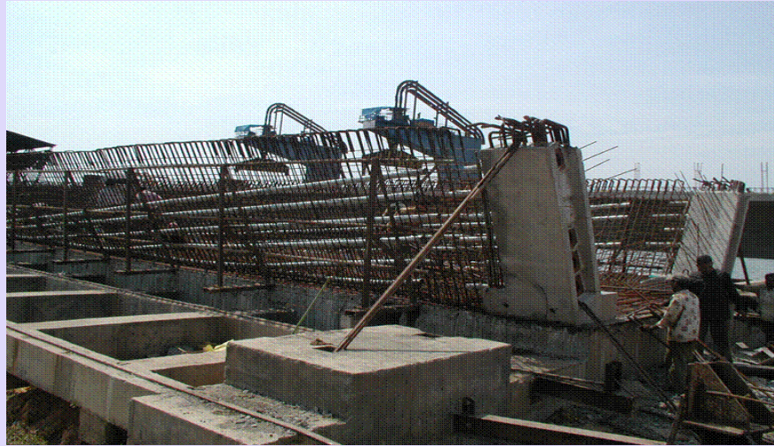
Figure 1-5.4 End-blocks in a bridge deck (Courtesy: Cochin Port Trust, Kerala)
