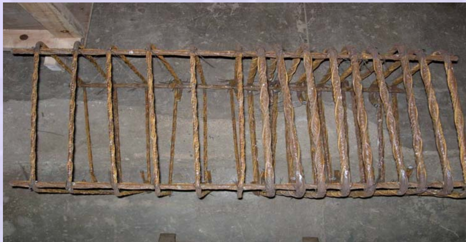
(a) Fabrication of end zone reinforcement
