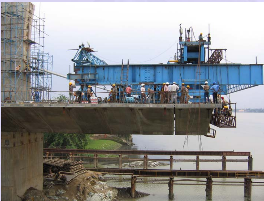
Figure 8-1.2 Segmental construction, Bridge over Hooghly, West Bengal (Courtesy: L & T Ramboll)
