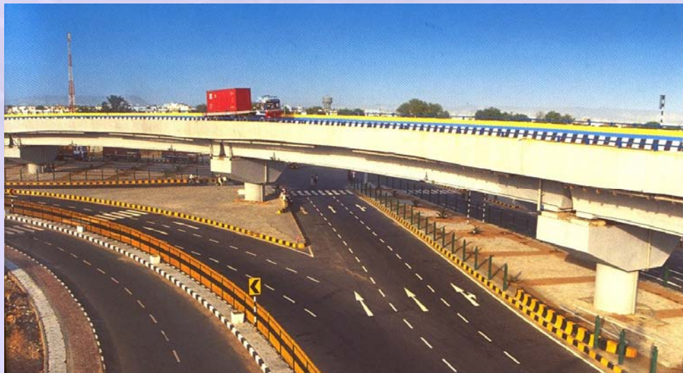
Figure 9-6.15 Curved box-girder bridge, Jaipur-Kishangarh Highway, Rajasthan (Reference: L & T Ramboll)
