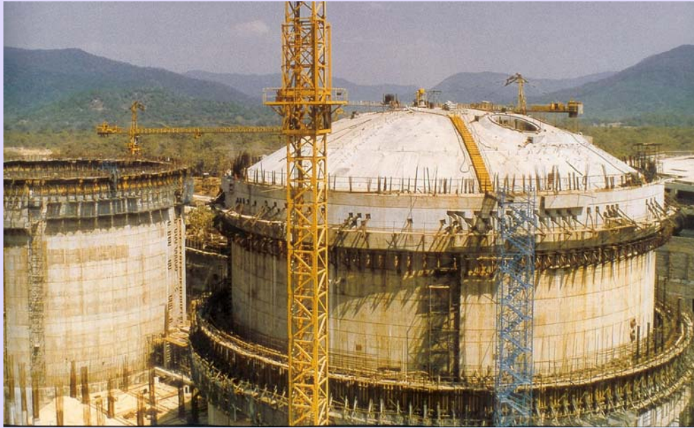
Figure 9-6.11 Containment Structure, Kaiga Atomic Power Plant, Karnataka (Reference: Larsen & Toubro)
