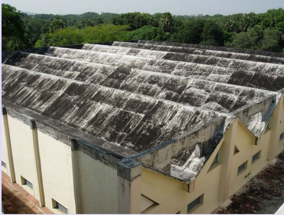
(a) Exterior view
